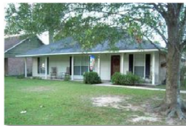
Typical ranch-style home in Central from the 1970s
